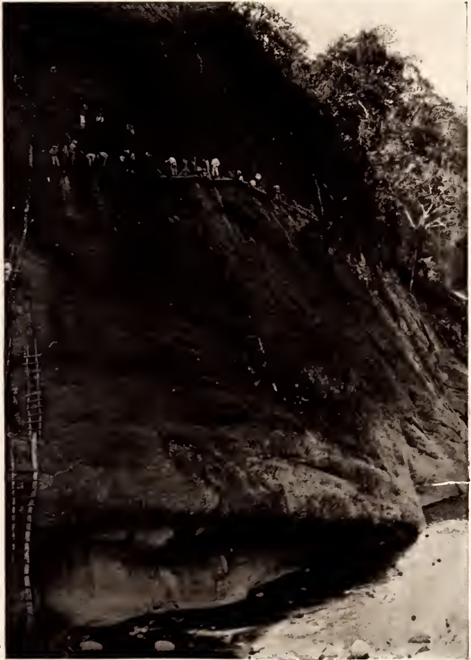
WORKING ON THE BENGUET ROAD.
